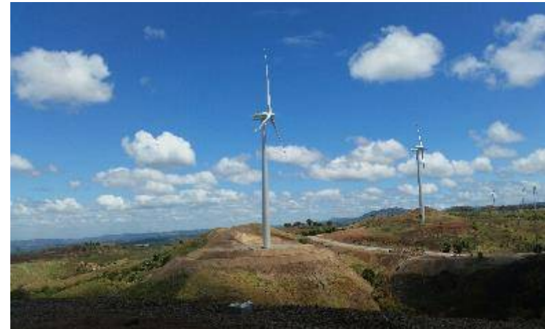
54 MW Rizal Wind Farm
