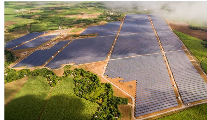
132.5 MW Cadiz Solar Farm
