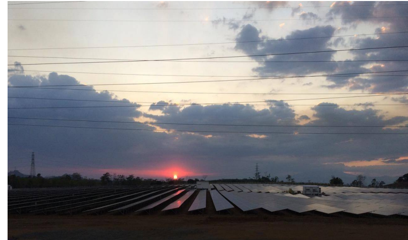
10.5 MW Kibawe Solar Farm
