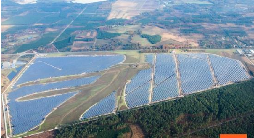
83.5 MW solar farm Arsac, France
